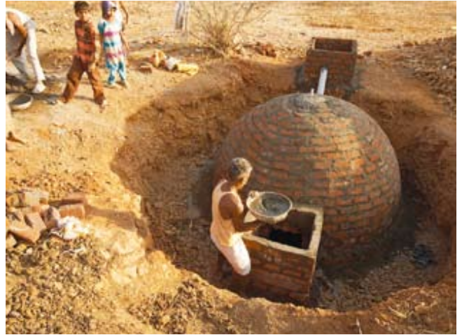
.... by constructing 150 biogas plants. As a greenhouse gas, the impact of methane is 21 times higher than CO 2 .
